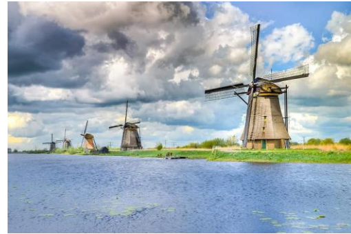
Horizontal axis wind turbine 14 th century – now
