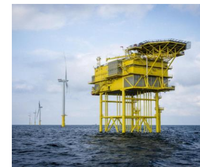
Offshore wind substation Source: offshorewindindustry.com
