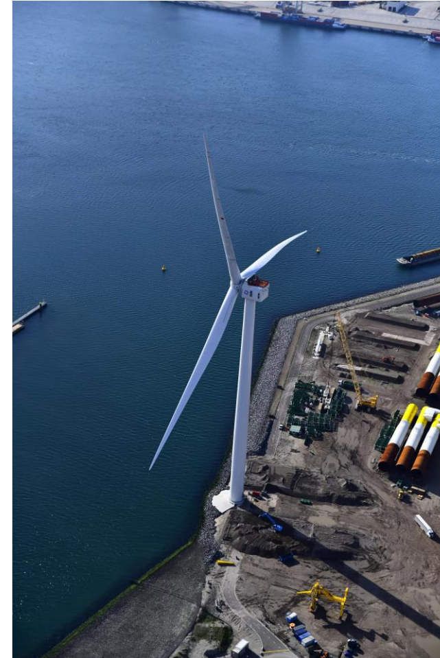
GE Haliade-X 12 MW wind turbine, Rotterdam Port.
