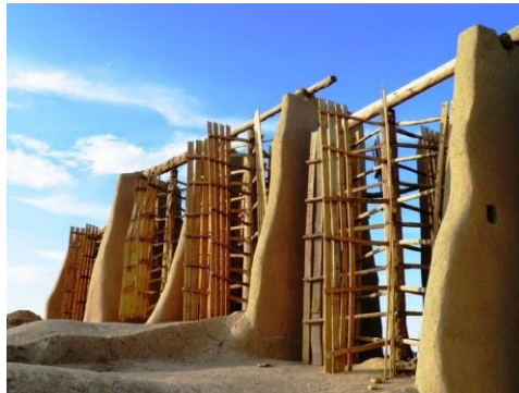
Vertical axis wind turbine, Panemone windmill, 700-900 AD
